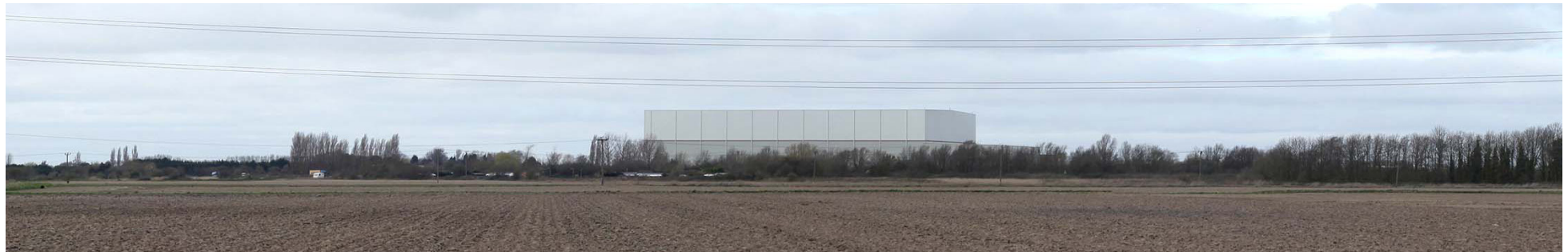
Photograph looking towards the cold store building
