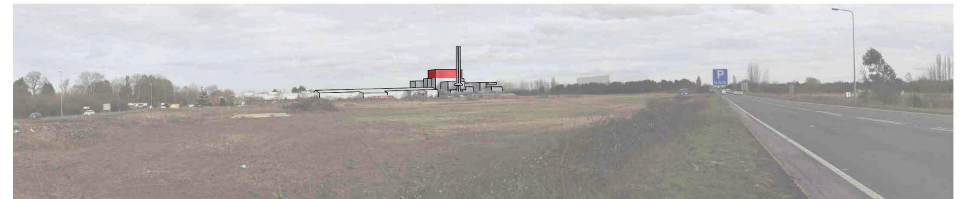
Highlighting key pedestrian view of the building (boiler house identified in red)
